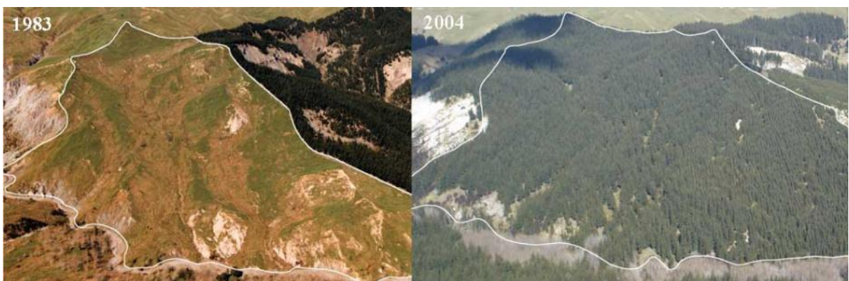
Figure 5: Active earthflow complex before (left) and after (right) reforestation. Rates of downslope earthflow movement declined by an order of magnitude within the period of a rotation of pines ~27-years (Marden, 2004).
