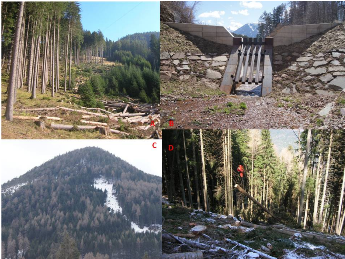
Figure 32 a, b, c, d: Italian observations: “edge-effect” cable harvesting (A); a substantial debris capturing structure (B); partial cut opening to enable natural regeneration (C) and cable harvesting corridor (D).
